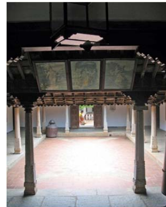
Fig. : Rural House at Kerla
